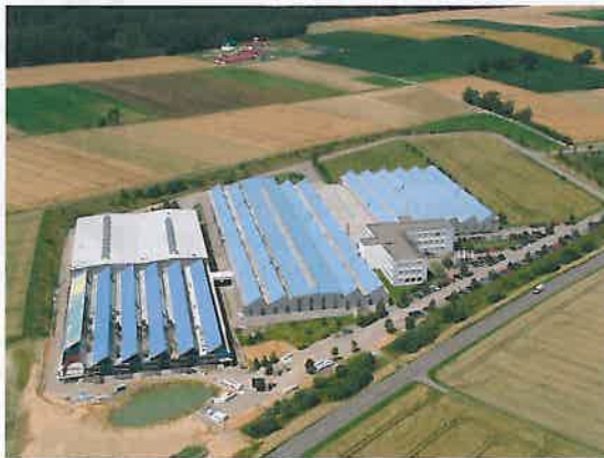
Fig. 1 The extended production facility from Paul (front) with the biomass power plant (back).
